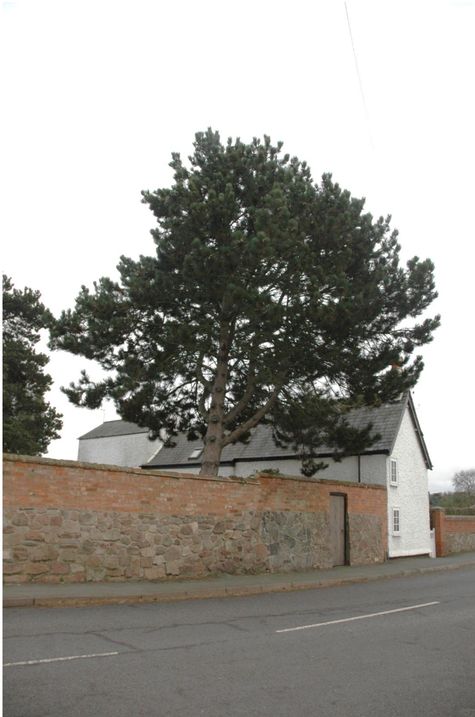
This is the pine at no 3 Soar Road and the reconstructed wall.
